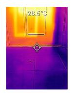
This image shows a laundry door with a draft stopper installed at the bottom. There is no heat entering the home as a result of this upgrade. The door also has a doggy door installed. Hotter temperatures can be seen around the perimeter of the magnetic door flap.
