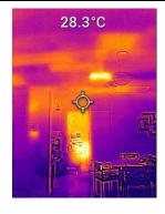
This image shows a lack of bulk insultation in sections of a living room roof cavity. A skylight above the table/dining area can also be observed. Heat gain or loss will occur in these zones leading to increased heating and cooling requirements and overall energy use.
