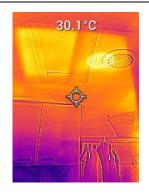
This image shows a roof hatch and extraction fan located in a laundry area. Roof hatches typically are easily removable to access roof spaces and cavities. Adding a layer of insultation to the top of the hatch would prevent heat from entering or escaping this area. Extraction fans can be fitted with top-hats to minimise heat loss from inside the home. These will automatically open via fan pressure when the fan is in operation.
